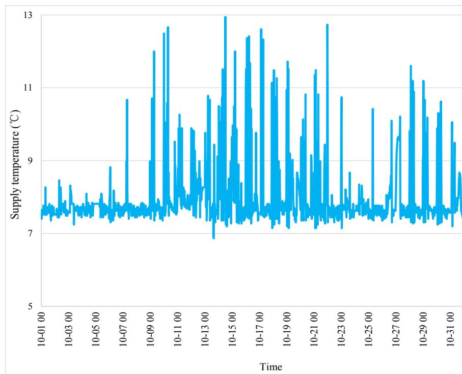
**Figure 7.** Actual supply temperature of the chilled water system.
