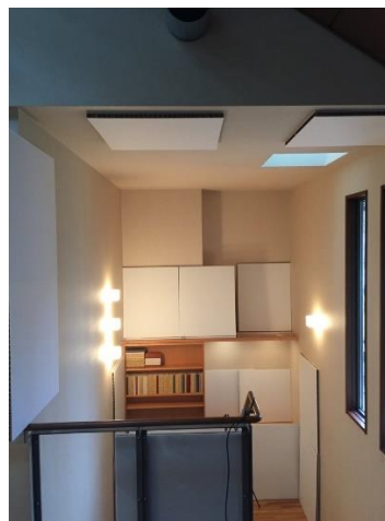
Figure 7. Sound absorption panel installation setup in the wall and ceiling of second floor.
