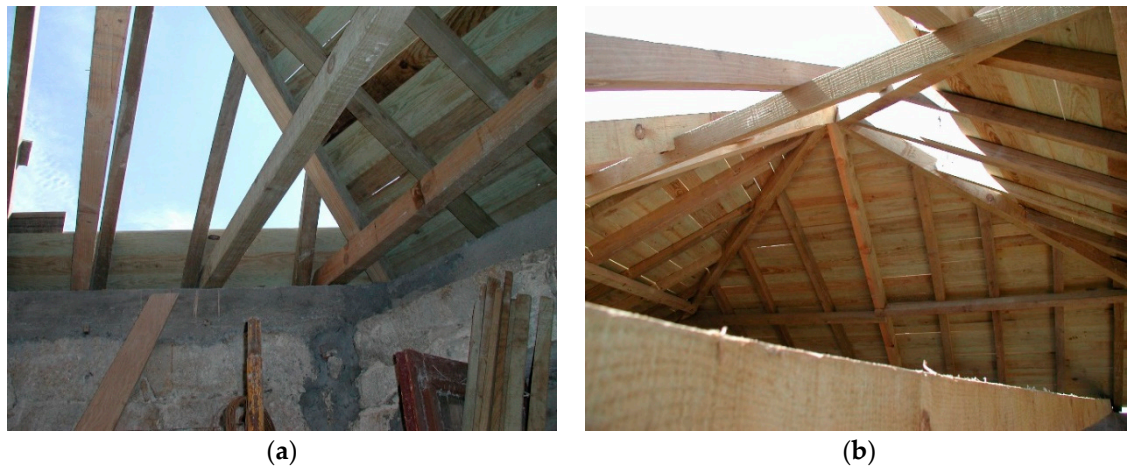
Figure 2. (a,b) Photograph of the hipped roof resting on party walls in Historic Center of Porto.
