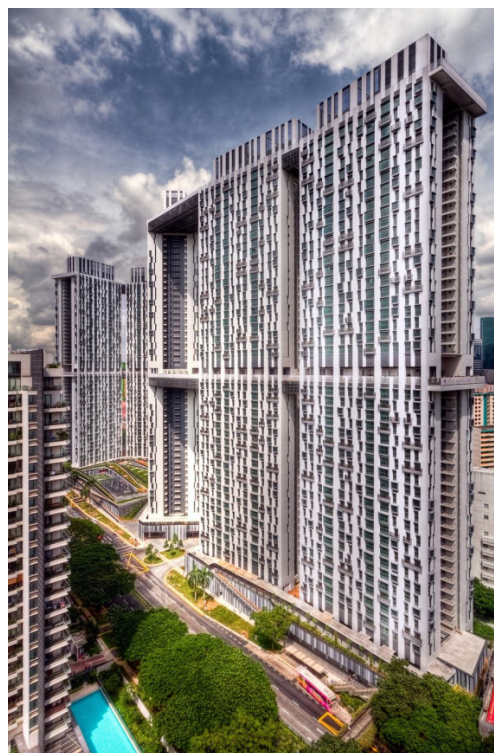
Figure 12. The Pinnacle@Duxton in Singapore is a major public housing project completed in 2009. It consists of seven 50-story connected towers. It supplies total of 1,848 units of 35 unit design variation. It was the recipient of the 2010 Best Tall Building Asia & Australasia Award by CTBUH [49].
