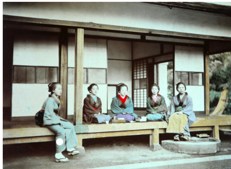
Figure 1. Adolfo Farsari. A peripheral transitional space featuring non- tatami flooring that mediates between the interior and exterior, while serving as both a circulation path and a drainage interface.
