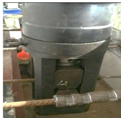
Figure 3. Process illustration of cold-extruded sleeve splicing for reinforcing bars.
