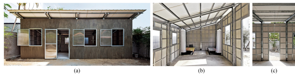
Figure 8. S-house 3. (a) Photograph of the facade of S-house 3, (b) interior photograph showing the exposed light-gauge steel framing, (c) photograph of the standardized light-gauge steel framing layout. Source: courtesy of Hiroyuki Oki.
