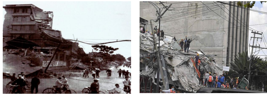
Figure 1. Actual damage diagram of concrete poles after the earthquake.
