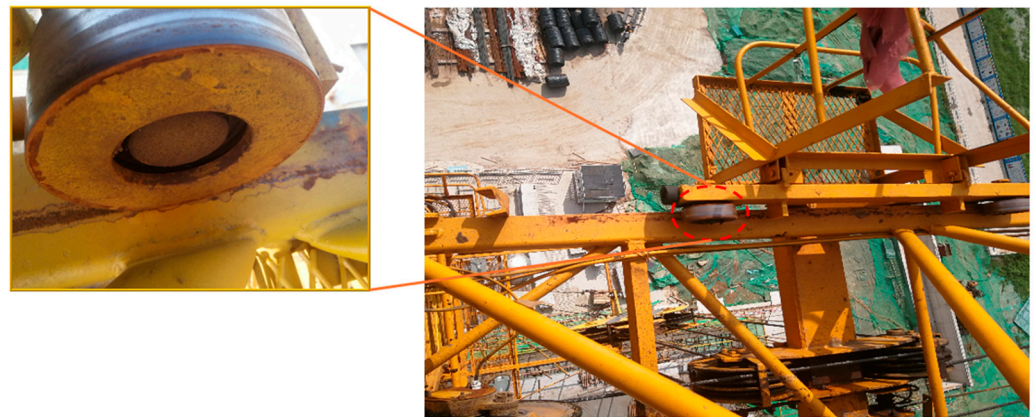
Figure 2. The contact between the luffing trolley and the jib.
