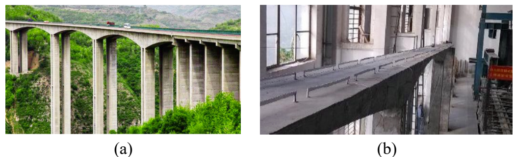
Figure 4. Heichonggou Grand Bridge (a), and its scaled model (b).
