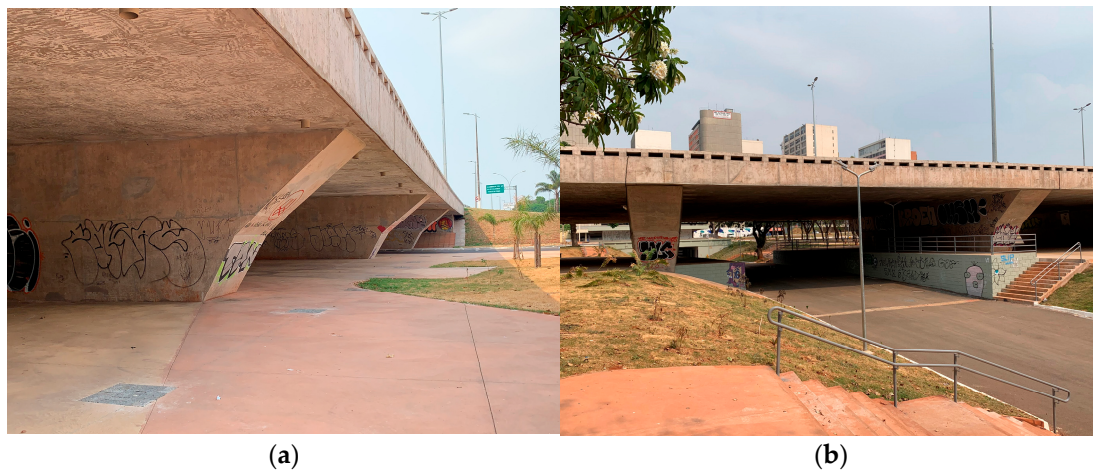
Figure 19. Viaduct after retrofitting: (a) view of the new jacketed column wall; (b) removal of the restaurant and integration with the new park.
