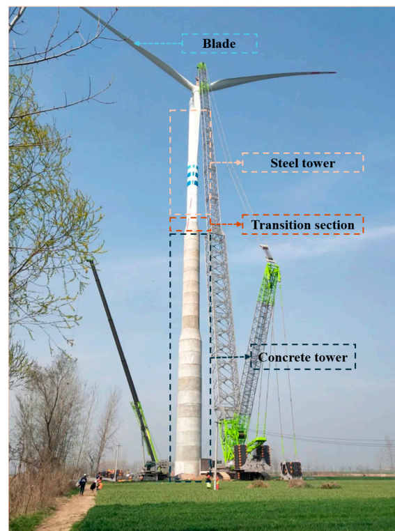
Figure 1. Steel-concrete hybrid wind turbine tower.
