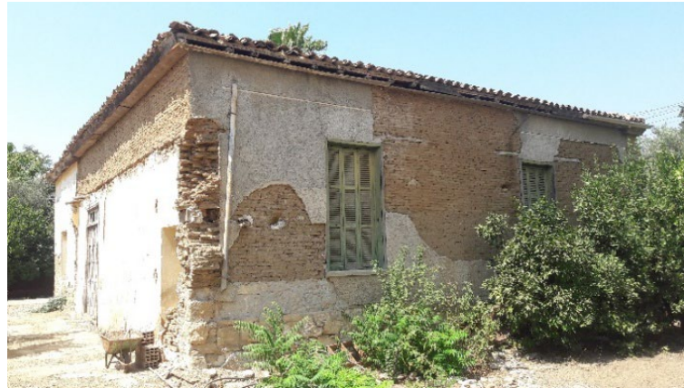
Figure 5. Visual examination of residential building in Nicosia, Cyprus.
