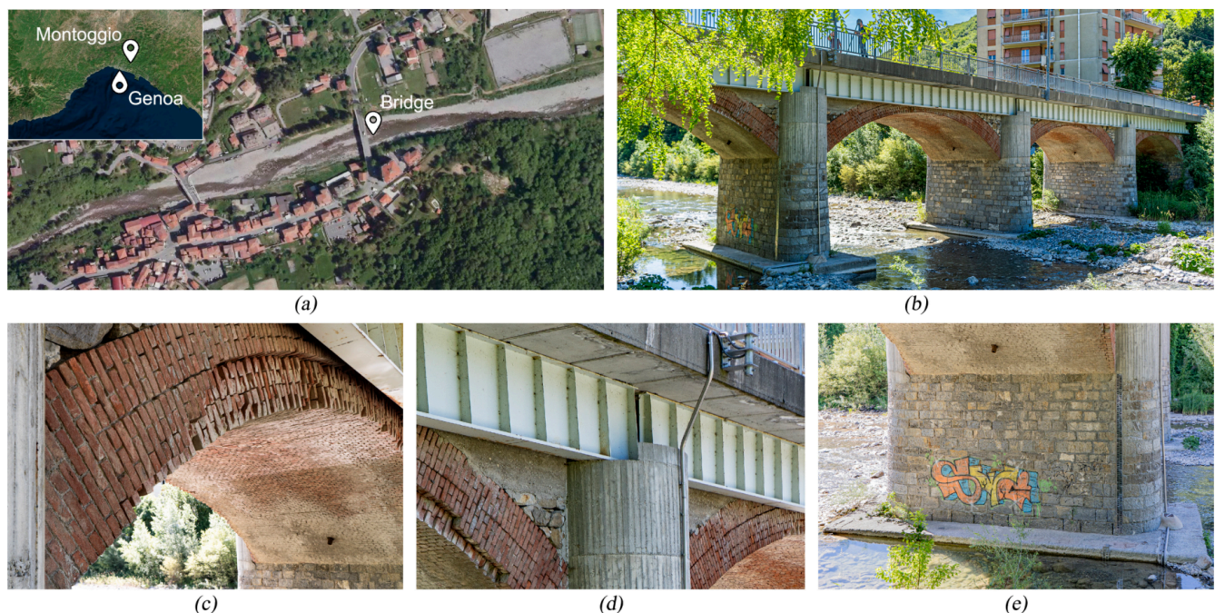
Figure 3. Photos of the bridge: (a) bridge location; (b) overall view of the bridge; (c) detail of one of the masonry arches; (d) detail of a pier showing the concrete retrofit, steel beam, and deck precast elements; (e) detail of the foundation.
