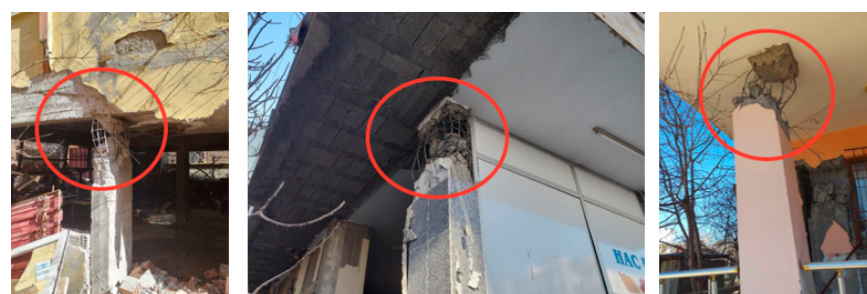
Figure 6. Representative failure modes observed at the upper confinement zone consequent to substandard transverse reinforcement detailing.
