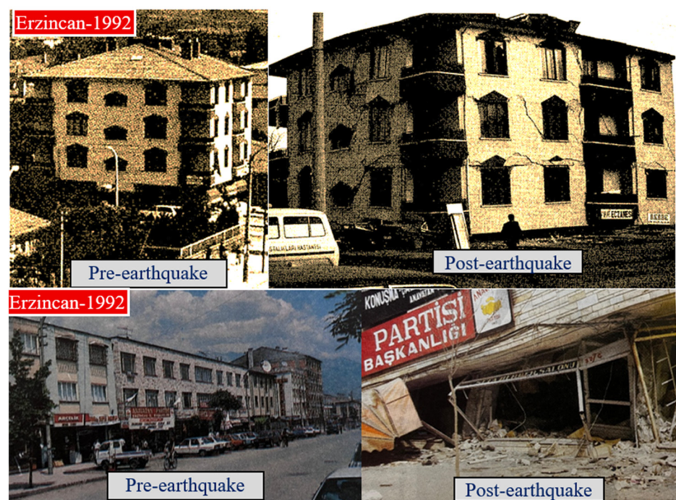
Figure 15. Examples of soft-story collapse mechanisms observed in reinforced concrete buildings in Erzincan Province before and after the 1992 earthquake.
