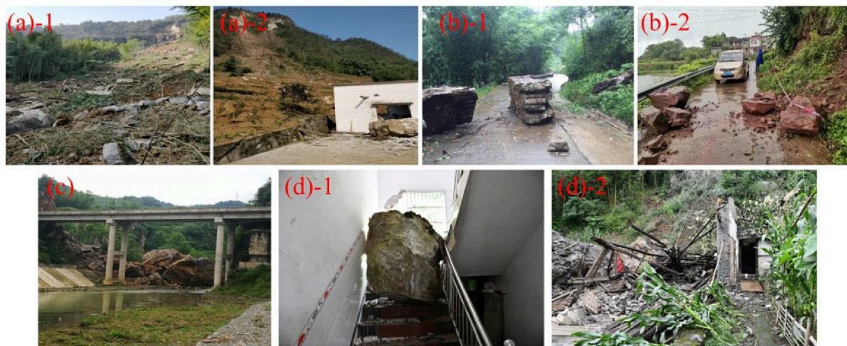
Figure 16. Seismic geohazards. (a)-1, (a)-2 Landslide. (b)-1, (b)-2 Road blocked by falling rocks. (c) River channel blocked by a landslide mass. (d)-1, (d)-2 Building destroyed by falling rocks.
