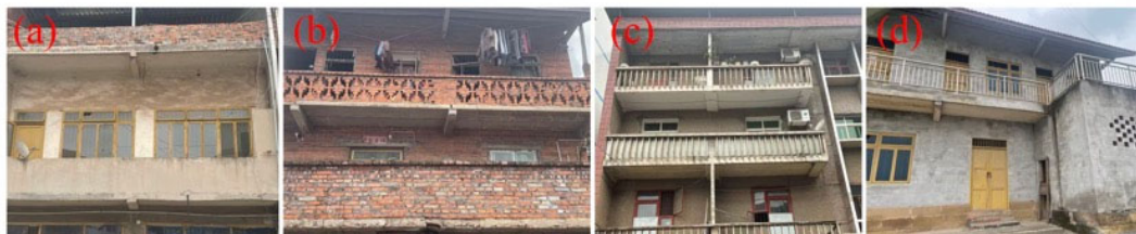
Figure 23. Different types of railing protective structures. (a) Solid brick masonry. (b) Hollow brick masonry. (c) Hollow precast concrete component. (d) Metal railing.
