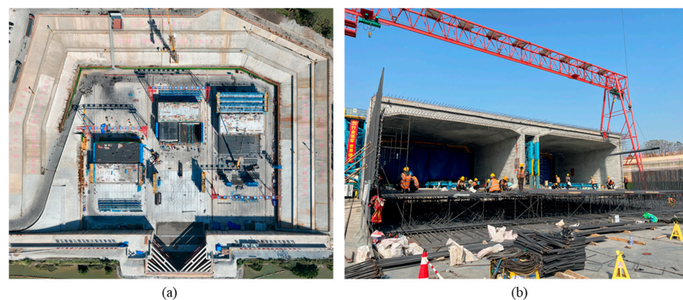
Figure 9. Site view of the experimental area and system deployment diagram. (a) Aerial view of the project dry dock site. (b) Actual scene at the experimental site.
