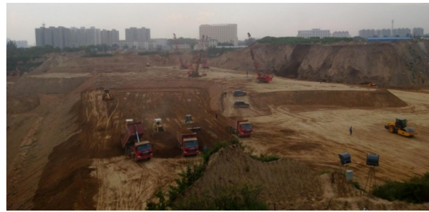
(a) Construction site photo of layered rolling.
