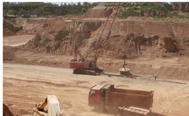
(b) Construction site photo of heavy tamping.
