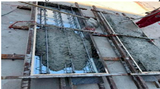
(c) Concrete pouring
