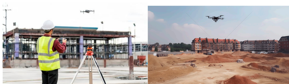
Figure 2. UAV monitoring of site violations on construction sites.
