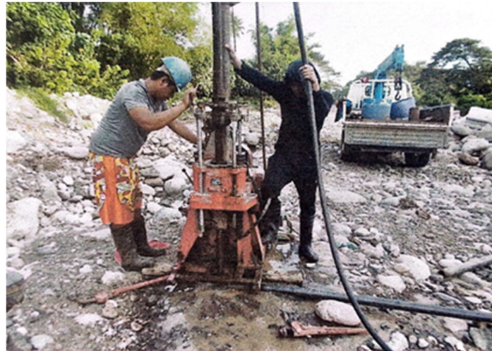
Figure 3. Field investigation setup showing the rotary drilling rig in operation using a water jetting mechanism.
