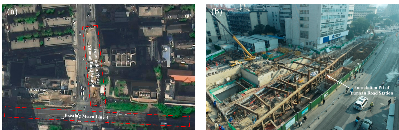
Figure 1. Location of the engineering project and the construction area. (a) Location of the foundation pit of Yunnan Road Station. (b) On-site construction of the foundation pit.
