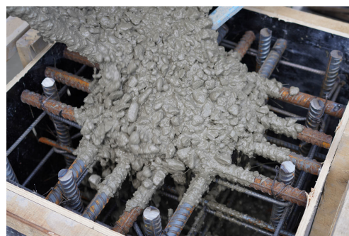
Figure 11. Accumulation during pouring.
