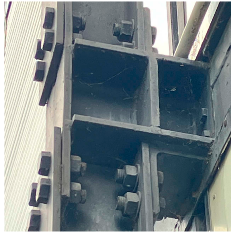
Figure 2. Beam-to-column joints of the main facade. Source: Upcycling Architecture in Italy. Design Workshop. Risultati/Results, 2024.
