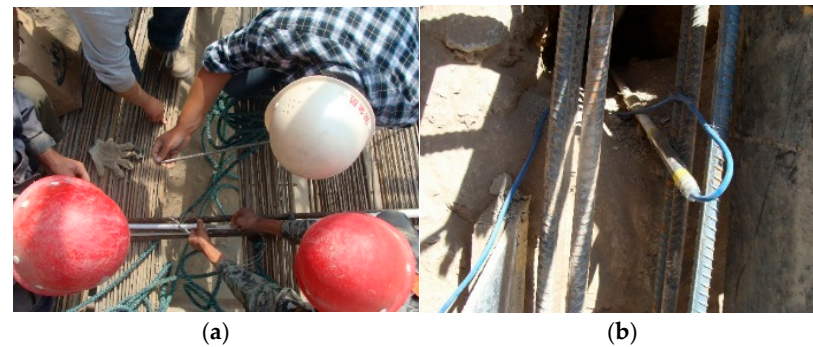
Figure 3. Field work: (a) on-site installation of metal-connecting rod; (b) the installation of displacement electric probe is completed.
