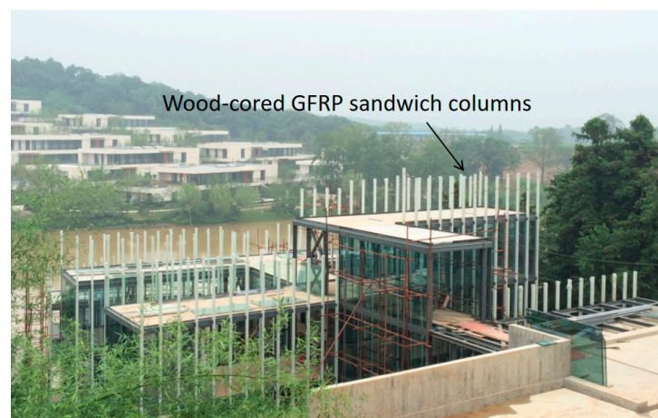
Figure 1. A tourism building, “Jade bamboo”, under construction using wood-cored GFRP sandwich columns in 2016.
