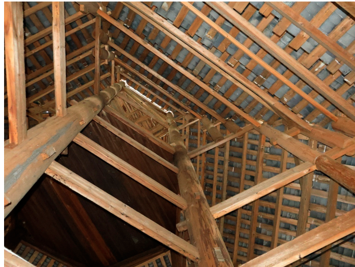
Figure 5. The interlocking structure of the tenon and mortise within the drum tower of Dali Dong Village. Photograph by the author.
