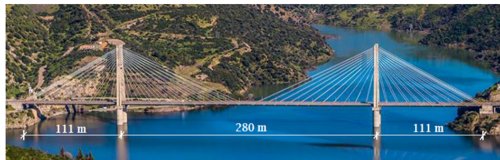
Figure 2. Elevation view of the Oued Dib Bridge.
