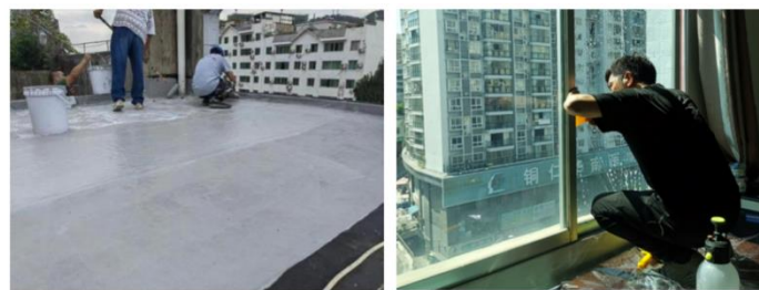
Figure 5. Construction site brushing the coatings and installing reflective films.
