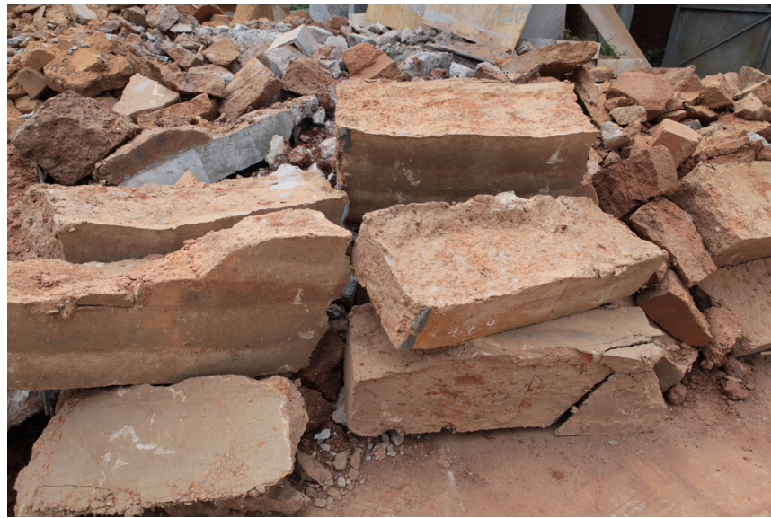
Figure 6. Blocks of a demolished RE wall.
