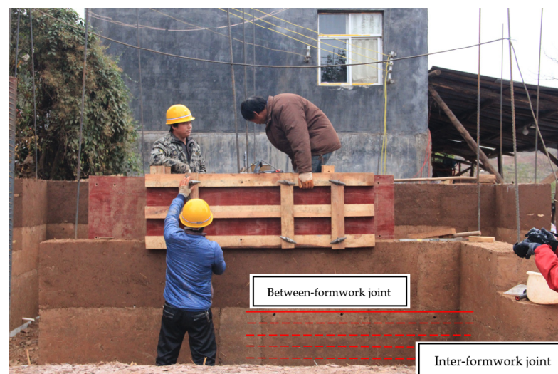
Figure 5. A unit of formwork.
