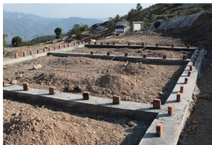
Figure 3. Anti-sliding key.
