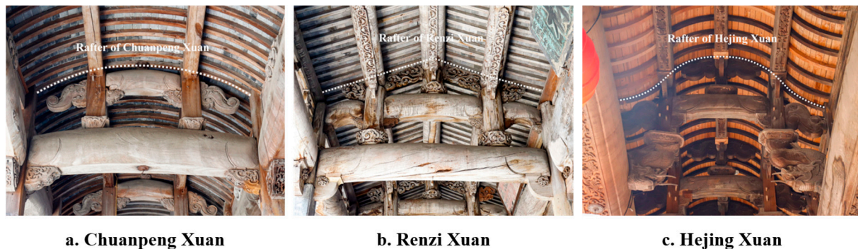
Figure 2. Types of “Xuan” and their rafters.
