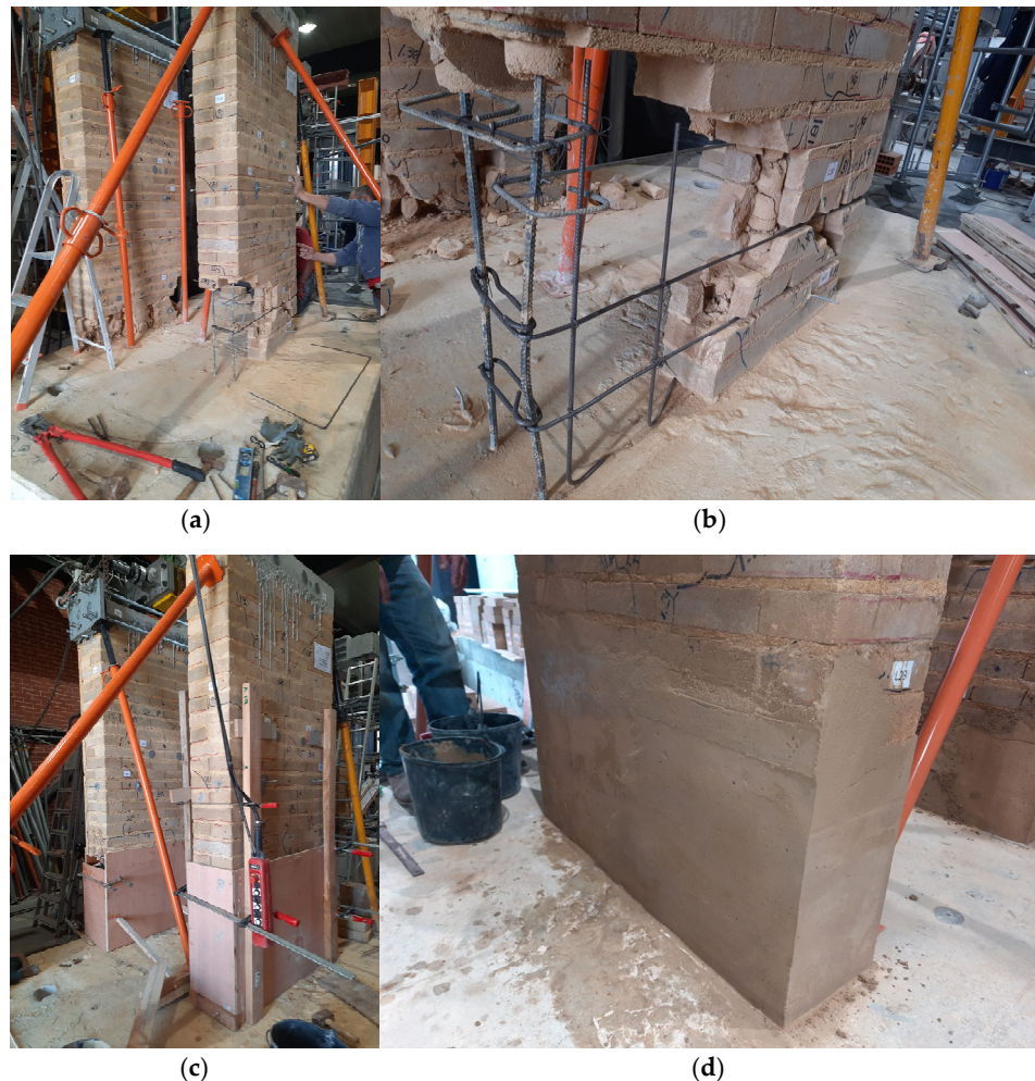
Figure 26. (a–d) C-wall recovery process.
