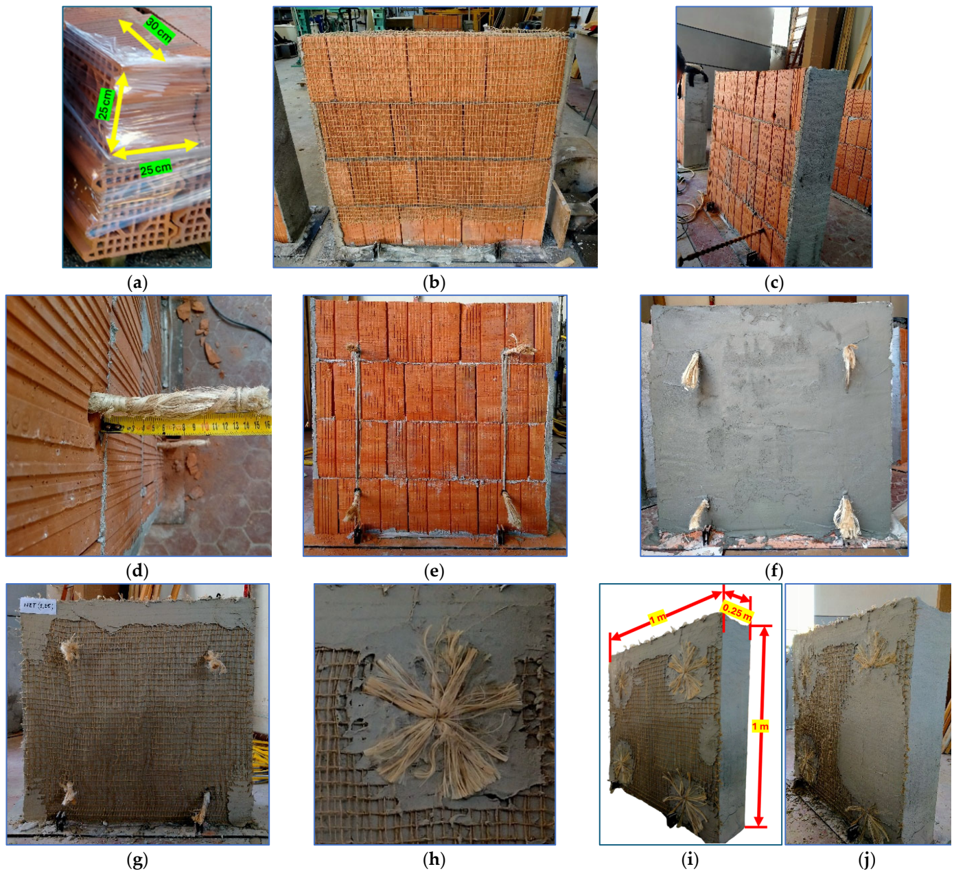
Figure 8. (a) Hollow bricks, (b) un-strengthened masonry wall before upgrading/retrofitting, (c) drilling of holes, (d) insertion of diaton, (e) application of liquid mortar, (f) first thin layer of mortar, (g) application net, (h) zoomed view of jute diaton, (i) fixing of all four diatons to the net, and (j) application of composite mortar.
