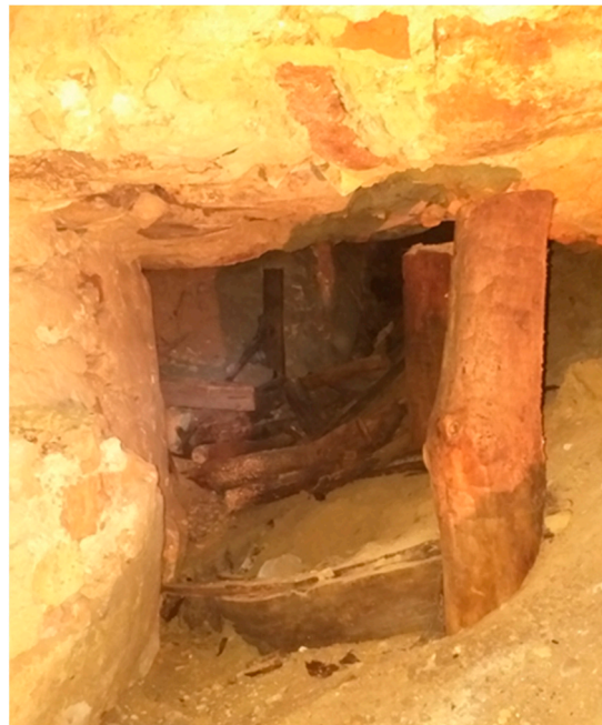
Figure 6. Rotten tunnel timber construction (authors' photo).
