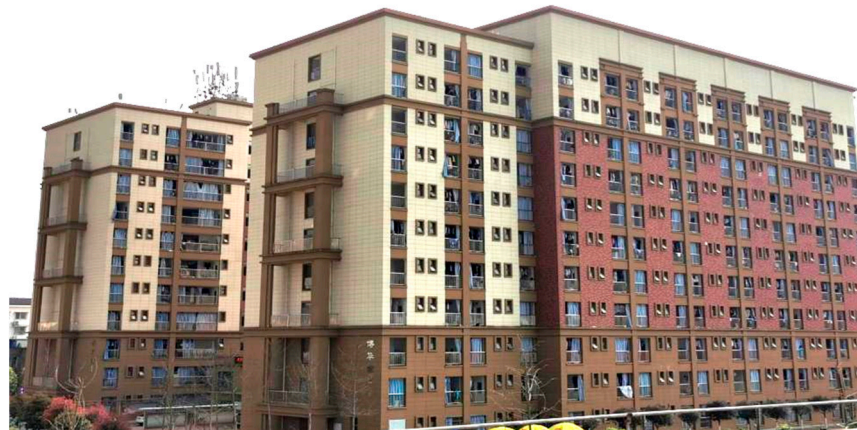
Figure 1. Actual View of Bohua Dormitory Building.
