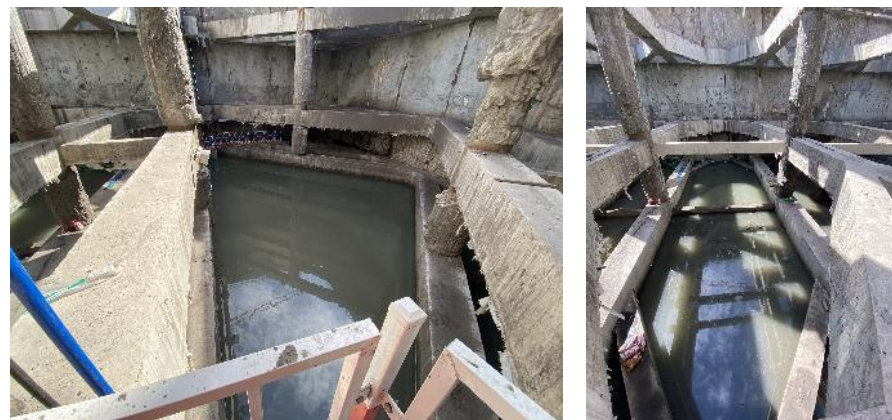
Figure 5. On-site water inflow condition at the foundation base.
