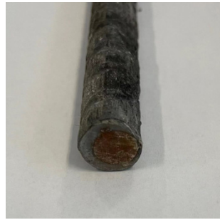
Figure 7. Misalignment of the inner steel bar.
