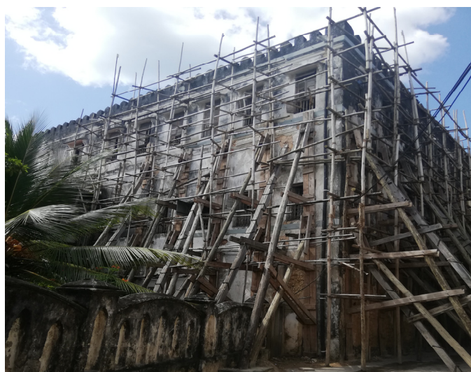
Figure 5. Example building renovation (photos by author).
