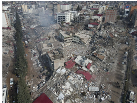
Figure 1. Kahramanmaraş after the earthquake.
