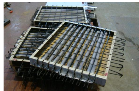
Prefabricated hollow floor slab
