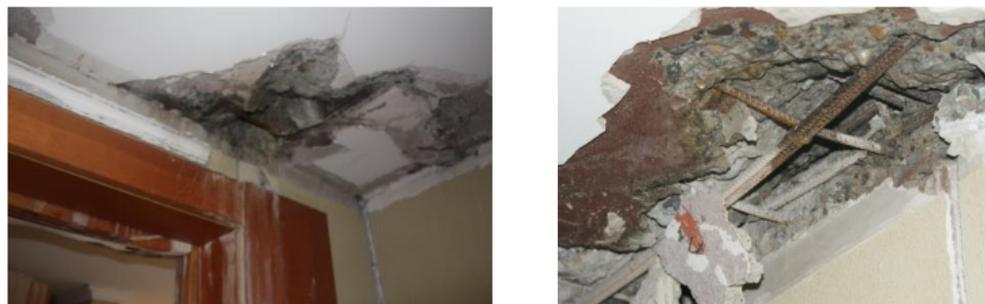
**Figure 15.** Slab S1. Damage in the first story.
