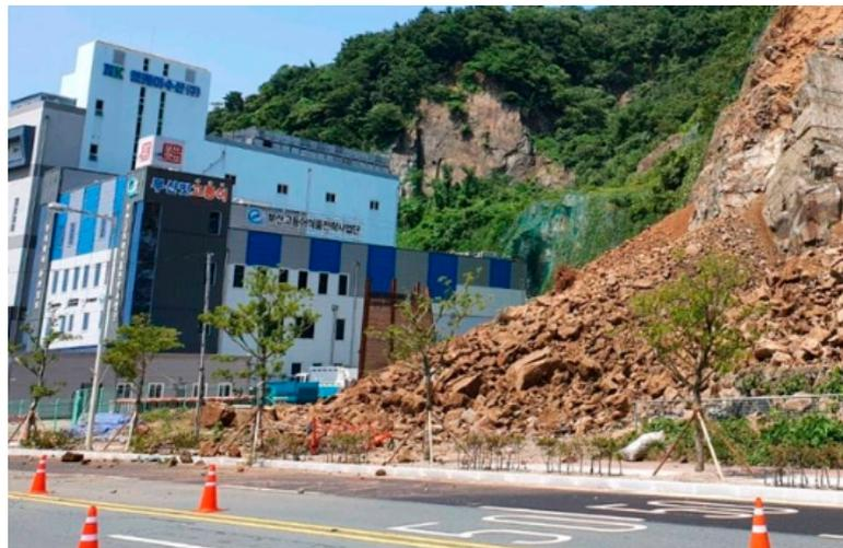
**Figure 2.** Building damage caused by weathering and scouring of soil slope in urban areas (Busan, Korea, 2021).
