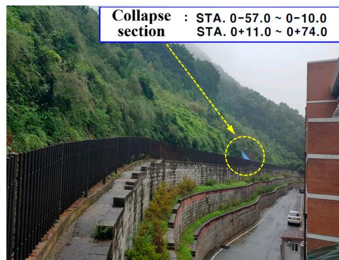
Figure 12. Slope failure site behind the high school building.
