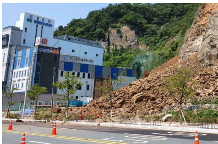
Figure 2. Building damage caused by weathering and scouring of soil slope in urban areas (Busan, Korea, 2021).
