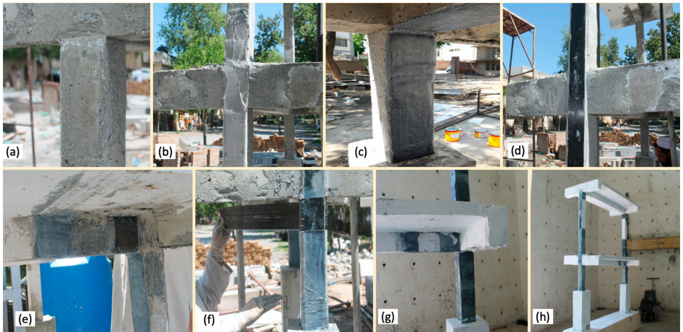
Figure 6. FRP application procedure (a) smooth concrete surface, (b) adhesive applied on the surface, (c) LCS installed, (d) CFRP laminate on the outer face of the column, (e) complete wrapping below joint, (f) complete wrapping around column, (g) view of strengthened joint, and (h) complete FRP strengthening scheme.
