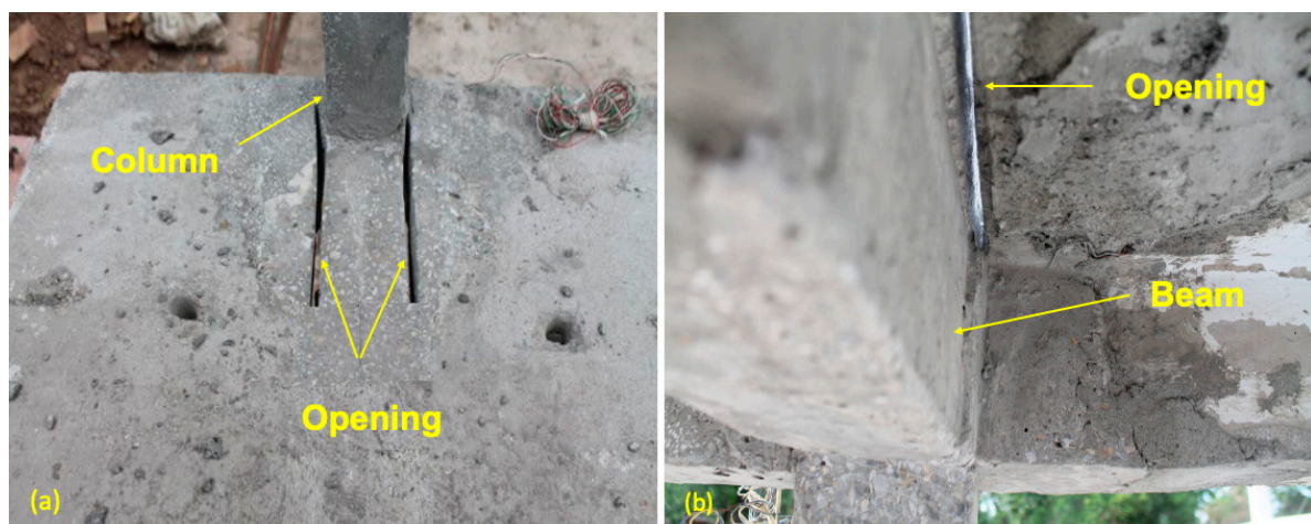
Figure 4. Opening in slab for aiding complete wrapping, (a) above joint and (b) below joint.
