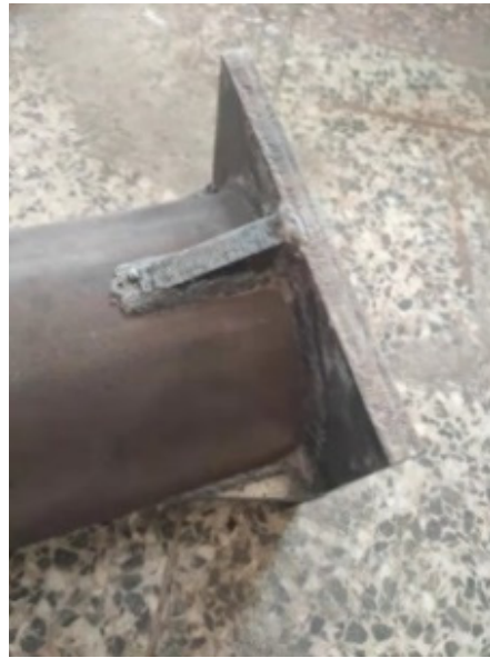
Figure 6. Completed welding stiffener.
