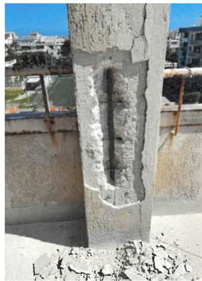
Figure 11. A column rebar before the extraction.
