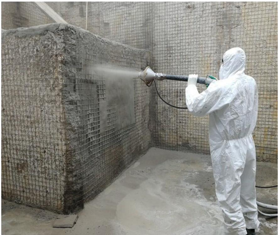
Figure 7. Field tests at a Voronezh construction site (private swimming pool).
