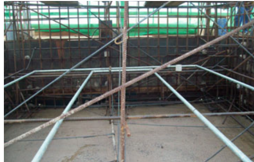
Figure 20. Post-cooling pipe installation on the spillway pillar of the Tocoma Hydroelectric Power Plant (photograph by W.P. Andrade).
