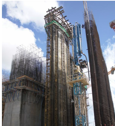
Figure 19. The construction of water intake pillars at the Tocomá Hydroelectric Power Plant, including the PI-04, which incorporates a framework.
