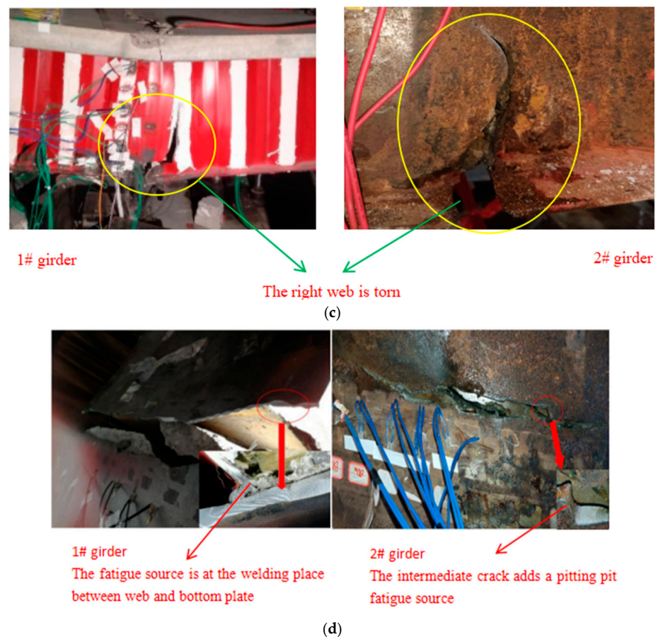
Figure 10. Test girder failure pattern and fatigue source. (a) Cracks at the bottom of the girder. (b) Cracks in the left web. (c) Right web crack. (d) Fatigue source.
